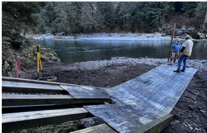
Steelheaders inspecting their work on the Wilson
